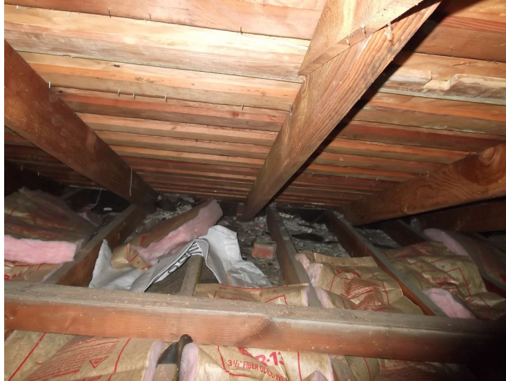
large area missing insulation
