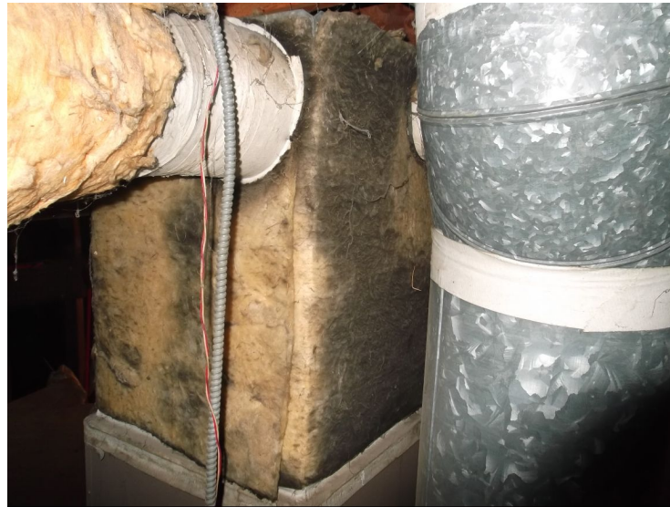
Darkened areas indicate excessive duct leakage
