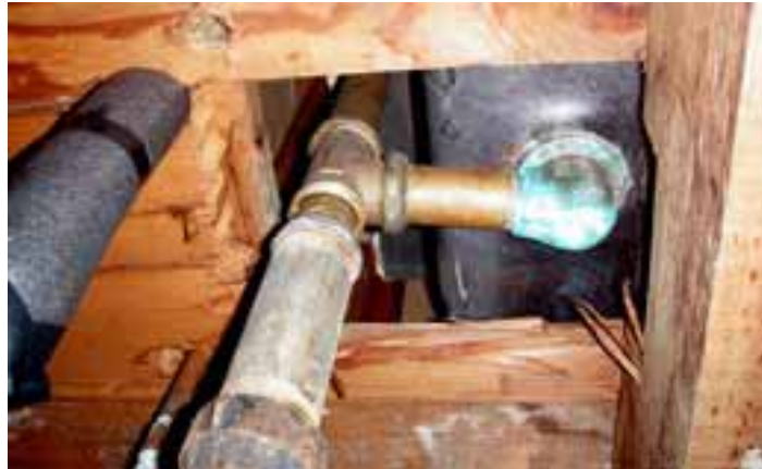
Before: Example of an unsealed hole.
