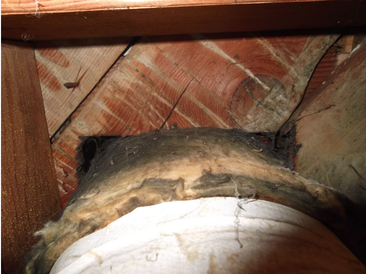
Hole in floor where duct enters house
