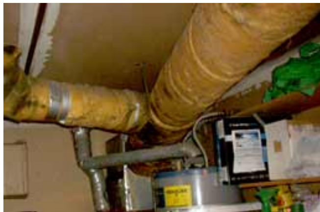
Before: A disconnected duct in your home.
