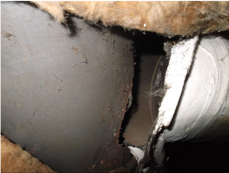
Large hole at connection to family room heating duct
