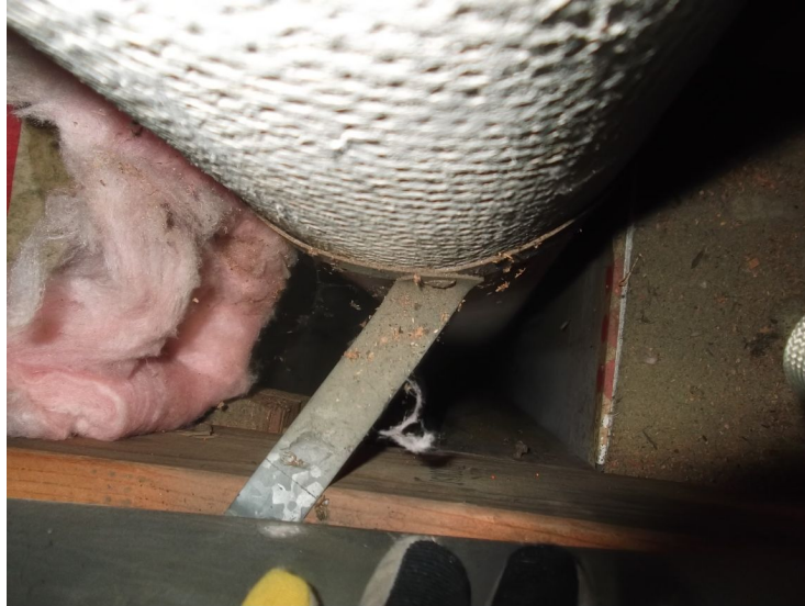
Hole in ceiling where flue exits into attic
