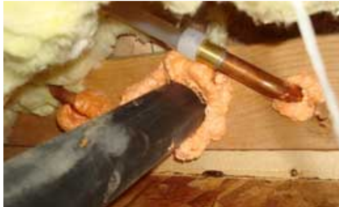
After: Example of a sealed hole.
