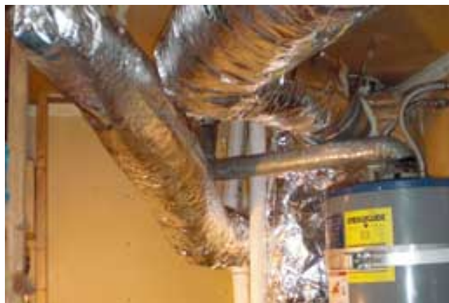
After: Triple sealed wireflex duct work.
