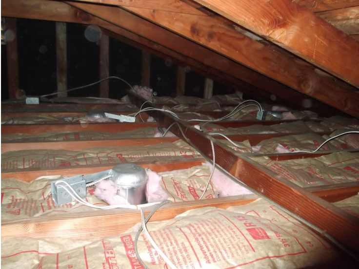
attic insulation is poorly installed and insufficient
